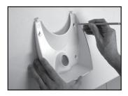
2. Using the bracket as a guide, mark the 4 wall holes with a pencil or pen.
