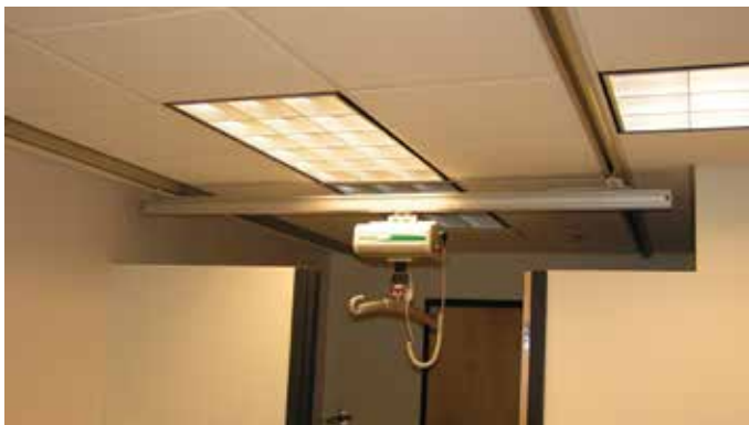
Lowered bathroom walls to allow the secondary rail to pass
